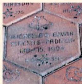
**FIGURE 3.** Fillers used in traditional engraving are subject to fading, oxidation, peeling, and separation.
